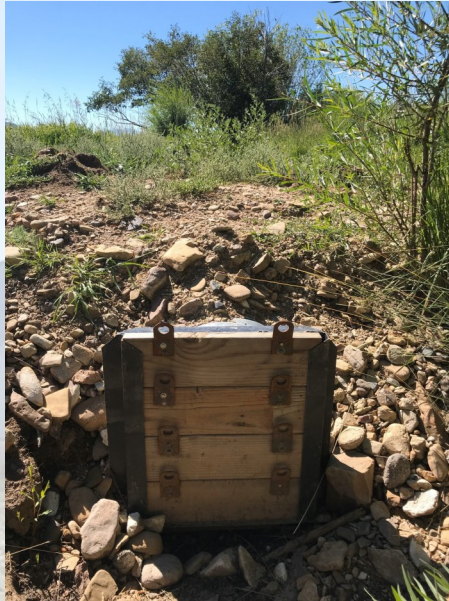
Irrigation Check & Turnouts
