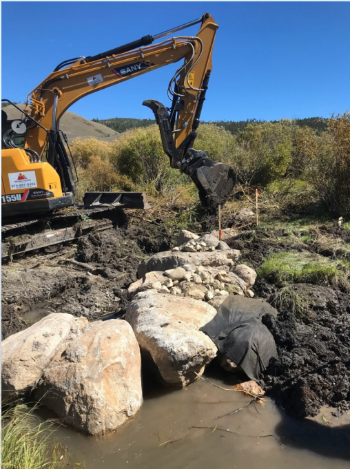
Irrigation Diversion Installation
