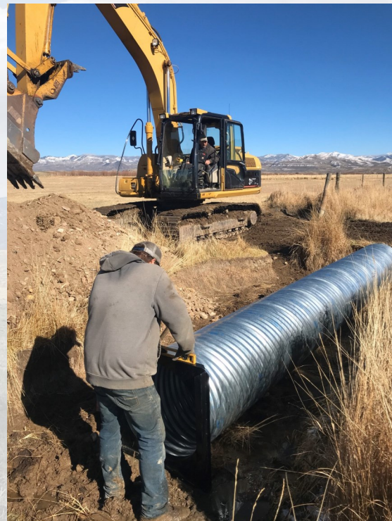
Irrigation Pipe Installation
