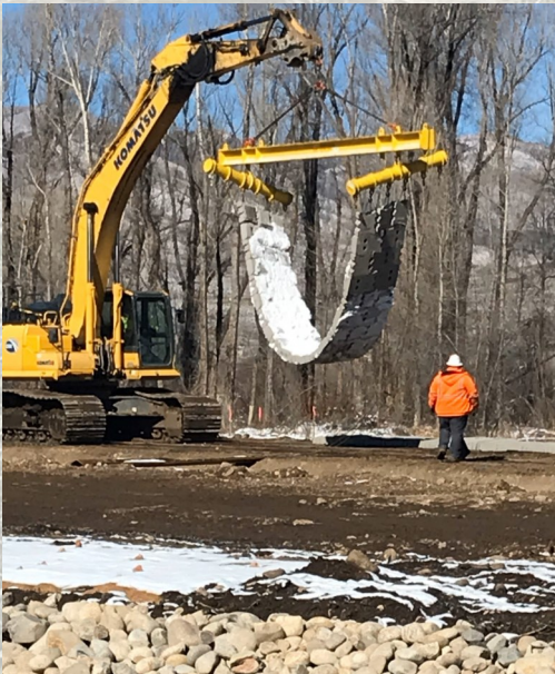
CO River Connectivity Channel
